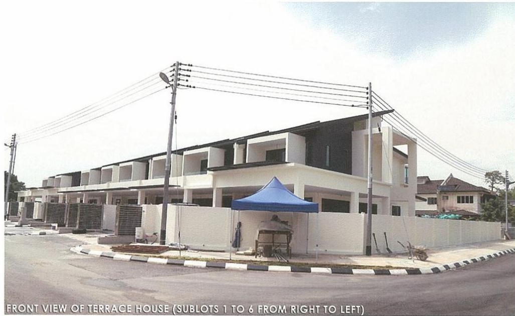
FRONT VIEW OF TERRACE HOUSE (SUBLOTS 1 TO 6 FROM RIGHT TO LEFT)
